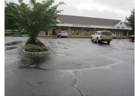
Pervious pavement can be installed at parking spaces adjacent to the building to capture and infiltrate runoff from the parking lot. A preliminary soil assessment suggests that the soils have suitable drainage characteristics for green infrastructure.
